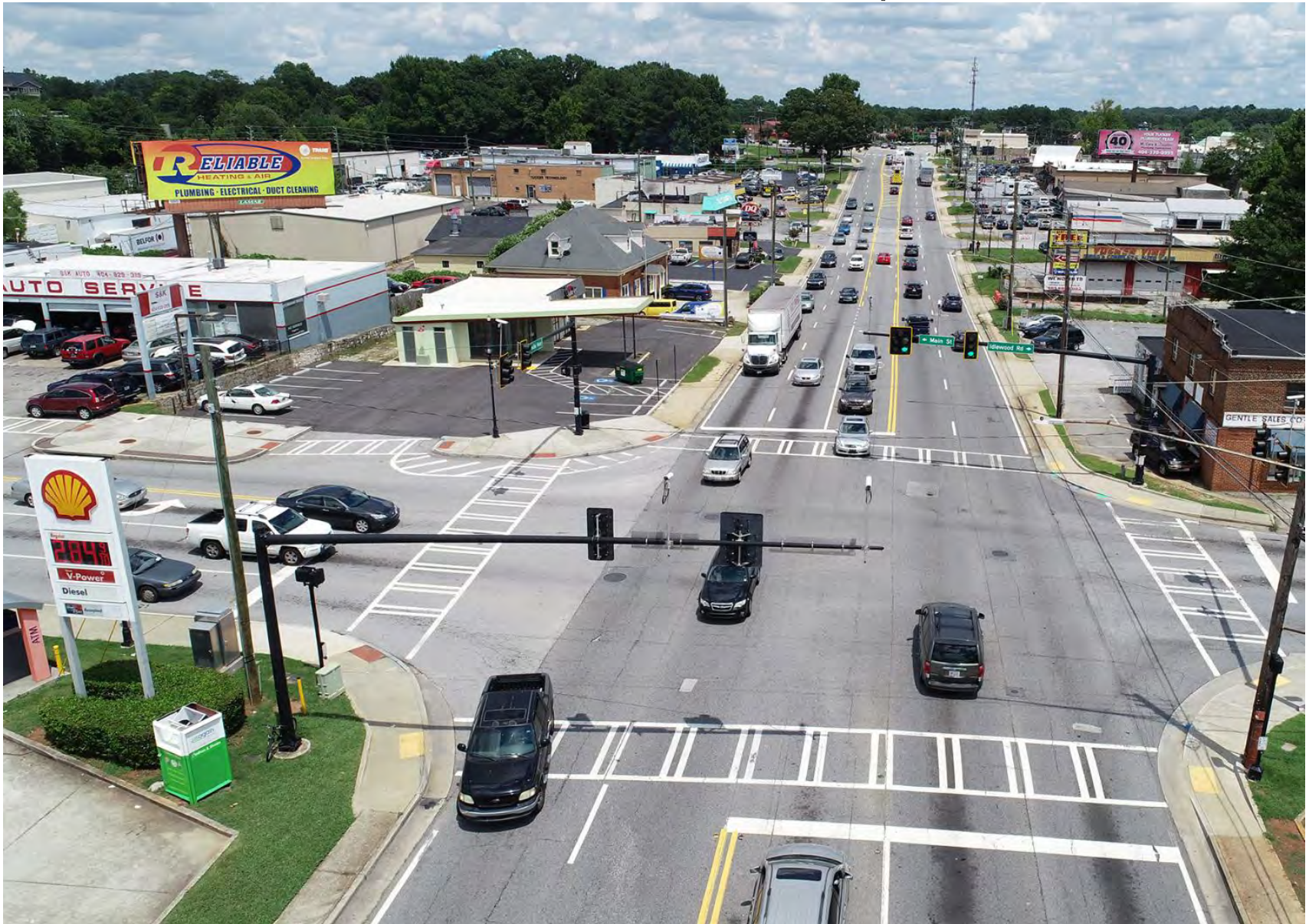
Lawrenceville Hwy Crossing - Before
