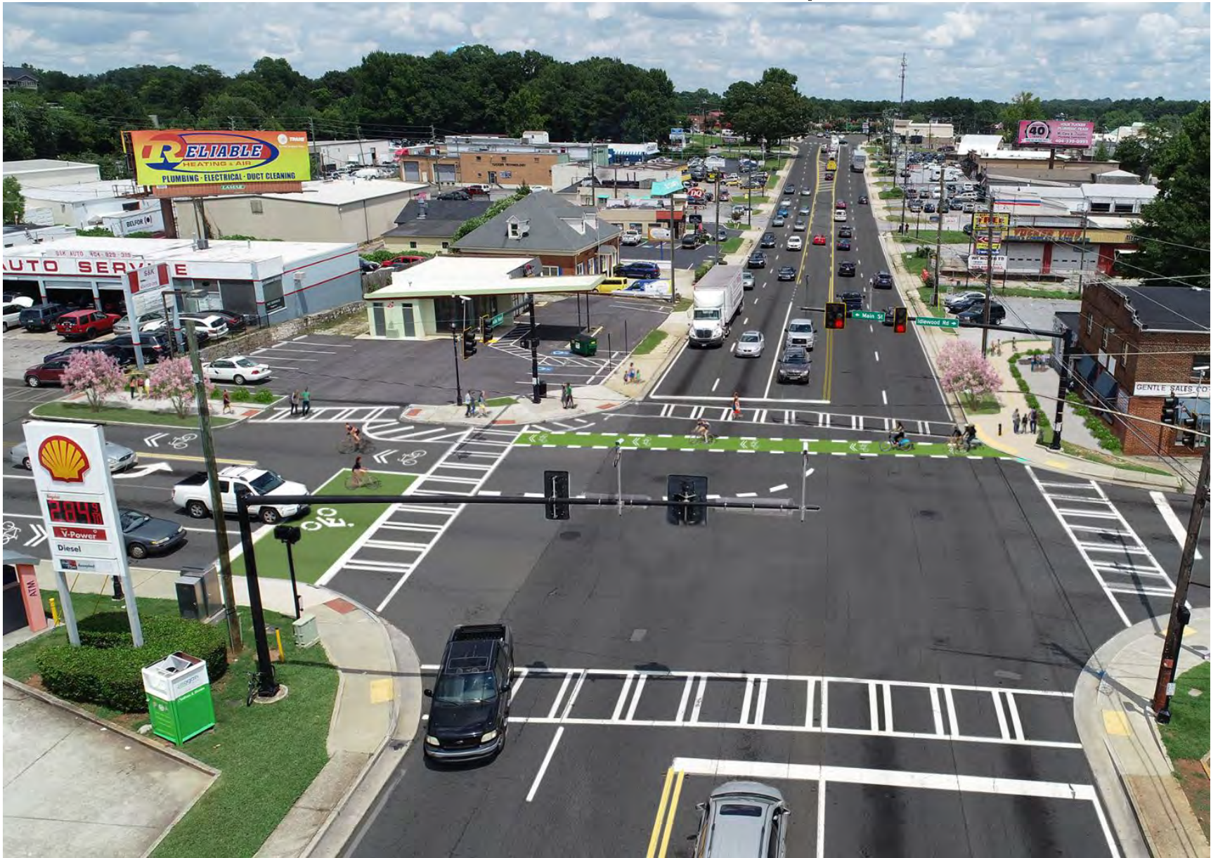
Lawrenceville Hwy Crossing - After
