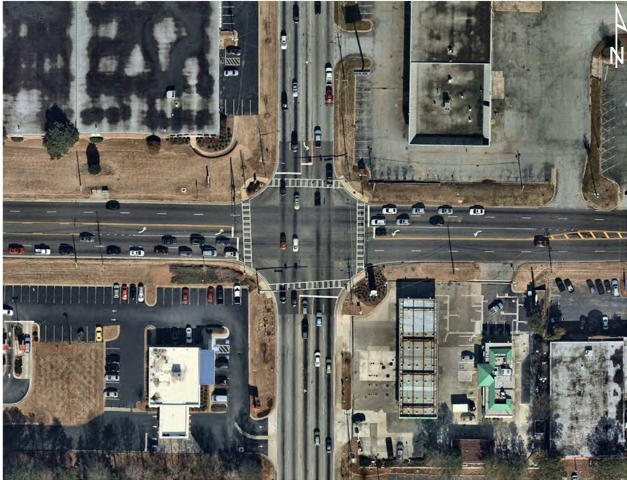
Figure 8: SR 236 at Mountain Industrial Blvd
