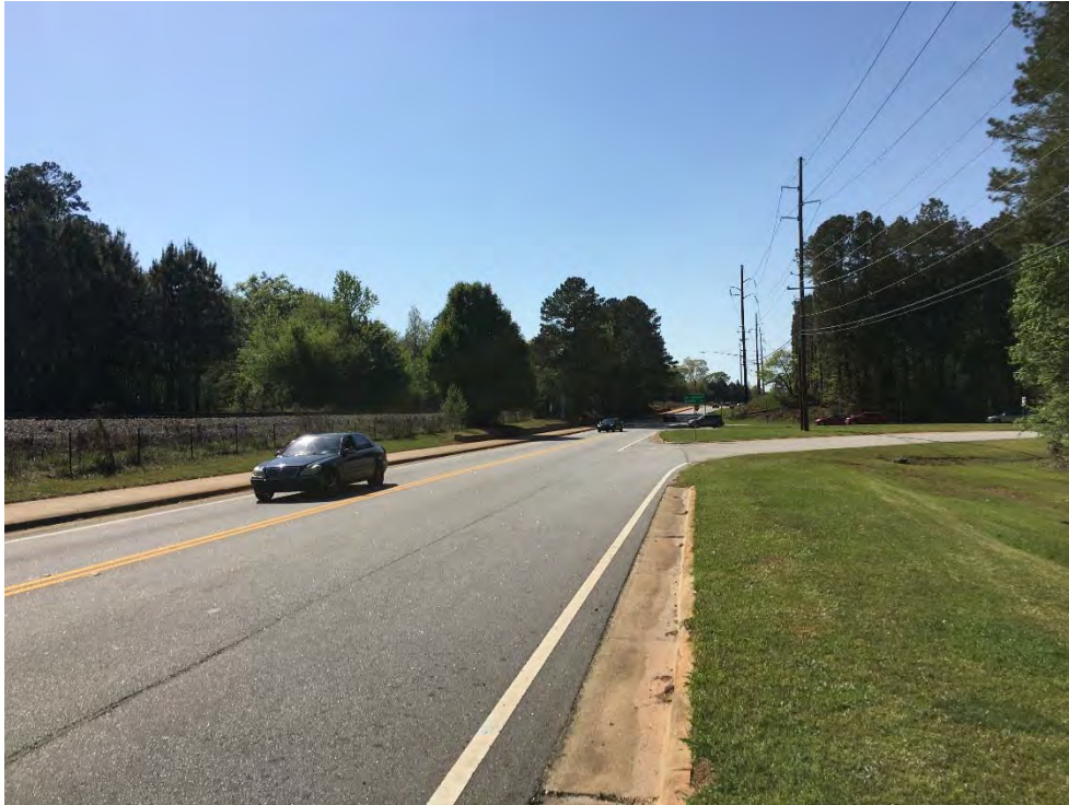
Figure A37: Westbound Approach to Southbound On-Ramp, SR 10 at East Ponce de Leon Avenue
