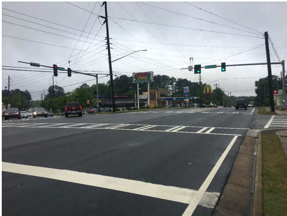
Figure A24: Westbound Approach, SR 236 at Montreal Road
