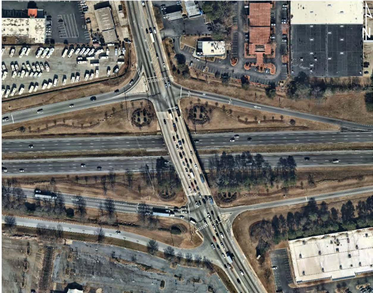
Figure 2: SR 410 at Mountain Industrial Blvd
