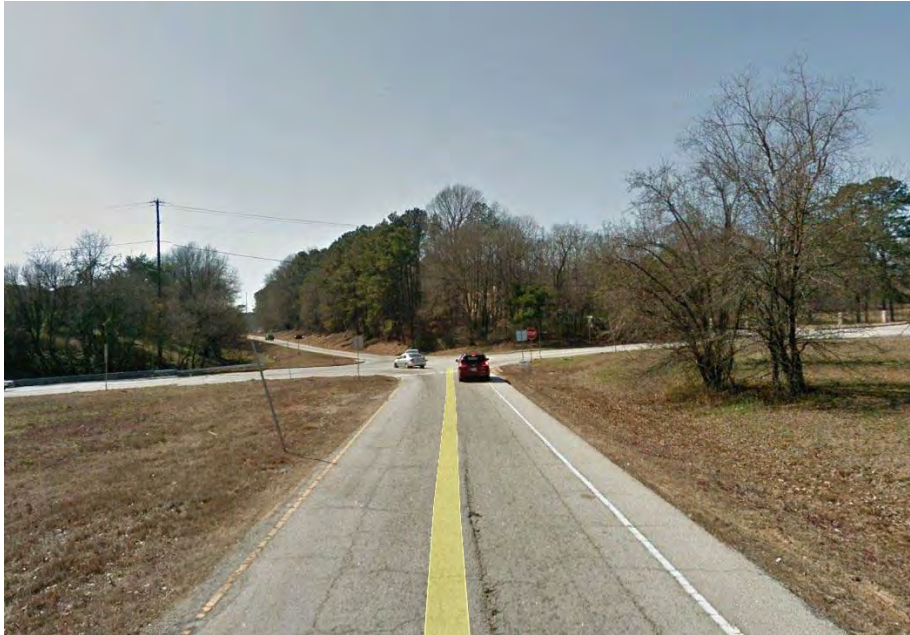
Figure A12: Westbound Approach, SR 410 at Brockett Road (North Intersection)
