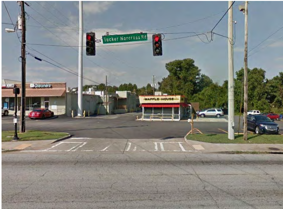
Figure A51: Westbound Approach, Tucker Norcross Road at Britt Road
