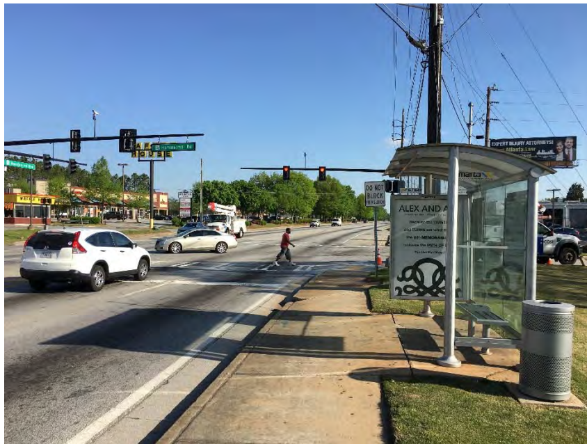
Figure A53: Northbound Approach, Mountain Industrial Boulevard at Hammermill Road
