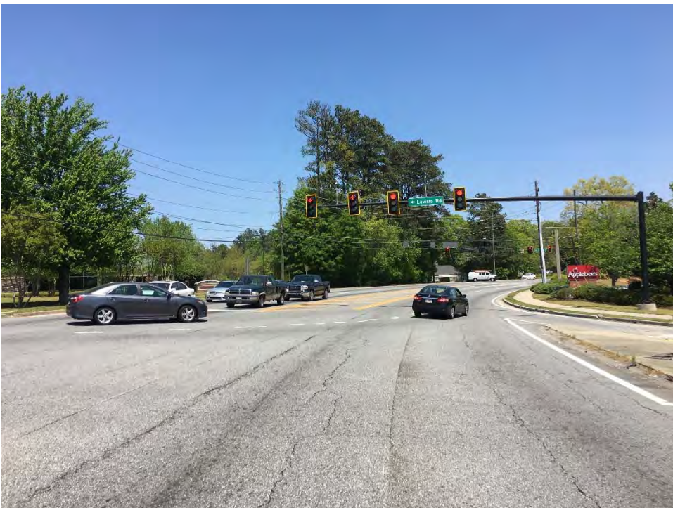
Figure A34: Northbound Approach, SR 8 at SR 236
