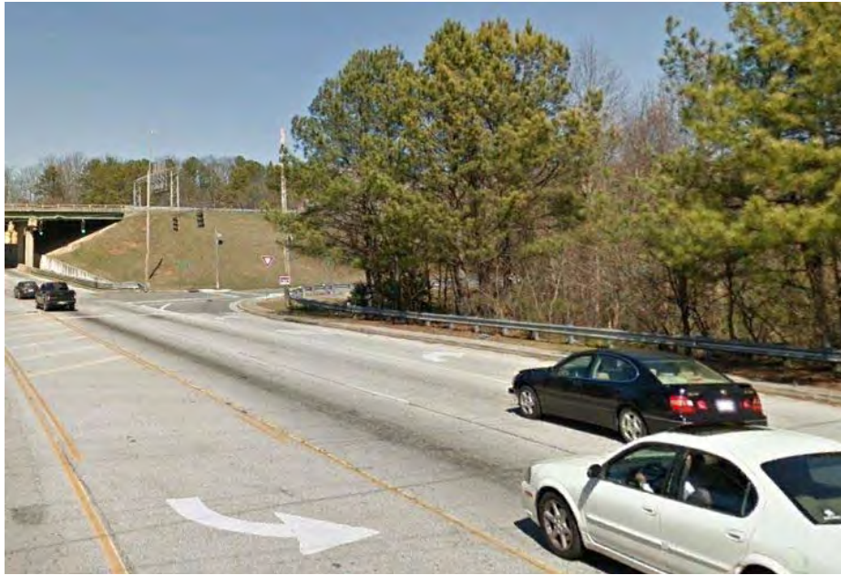
Figure A9: Northbound Approach, SR 410 at Brockett Road (South Intersection)
