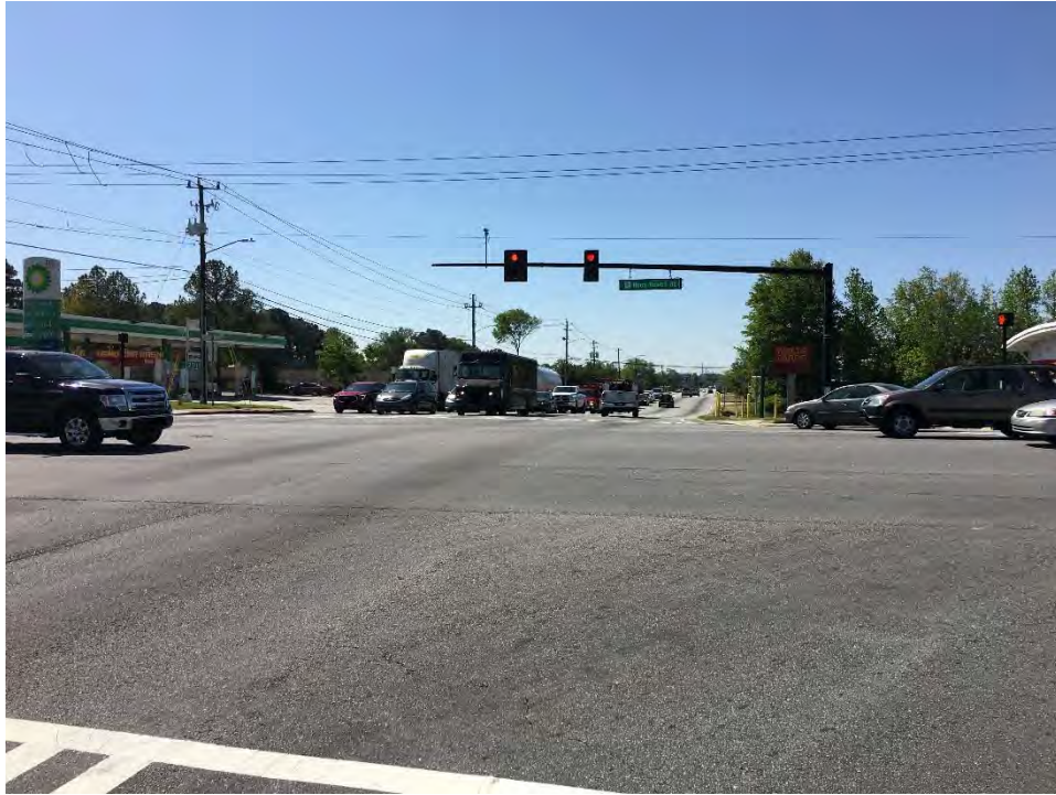
Figure A19: Southbound Approach, SR 236 at Mountain Industrial Boulevard
