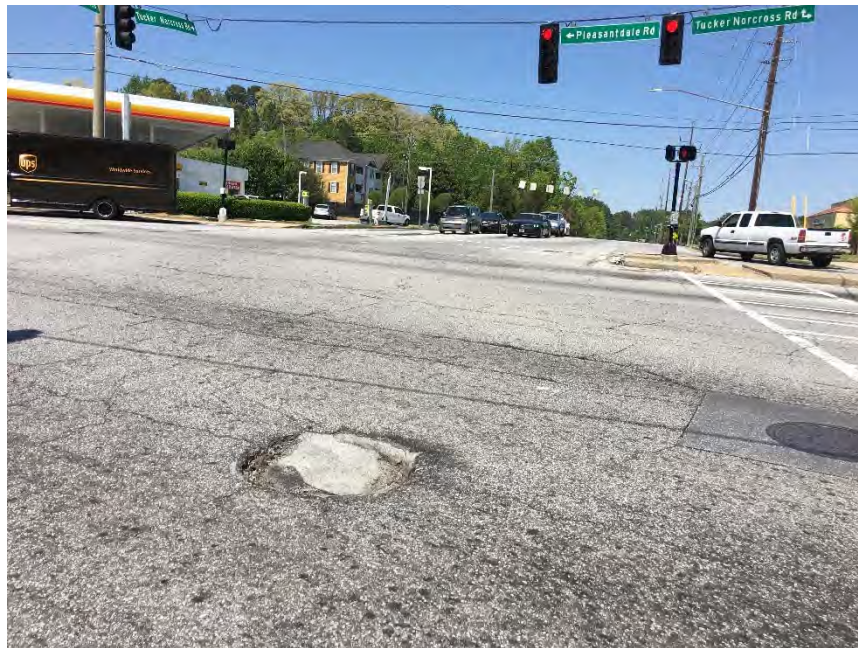
Figure A62: Eastbound Approach, Tucker Norcross Road at Pleasantdale Road
