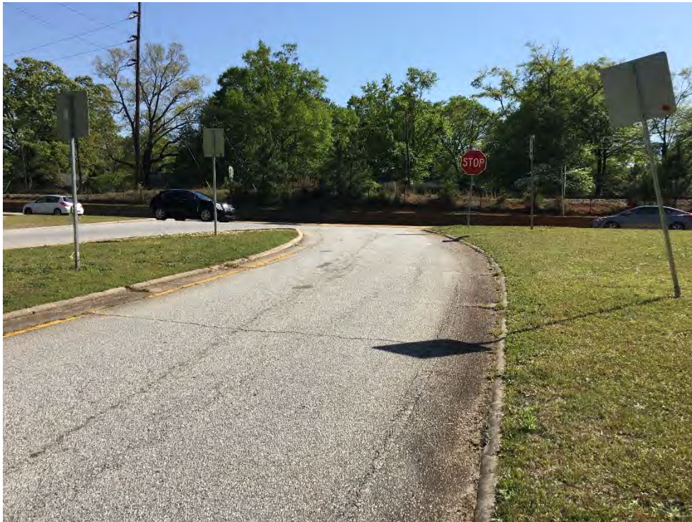
Figure A38: Northbound Approach Off-Ramp, SR 10 at East Ponce de Leon Avenue
