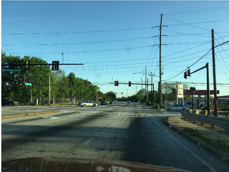
Figure A47: Northbound Approach, Mountain Industrial Road at East Ponce de Leon Avenue
