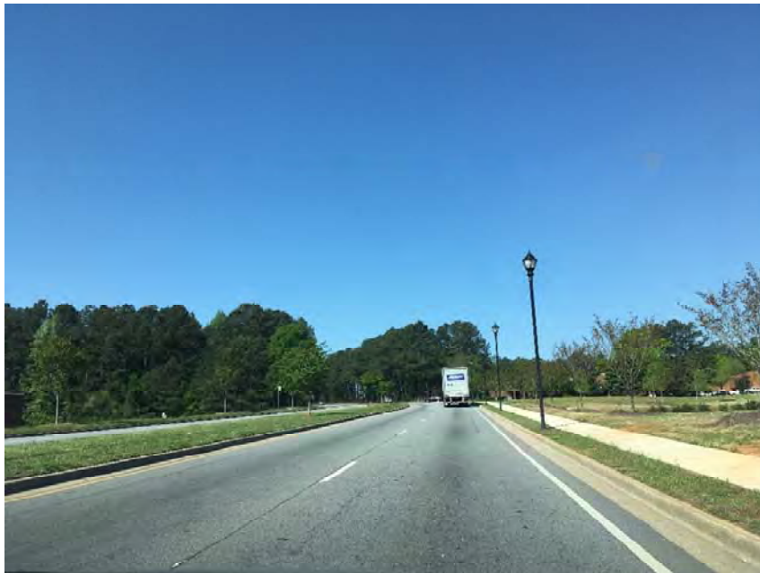
Figure A77: Westbound Approach, Mountain Industrial Boulevard at Tuckerstone Parkway
