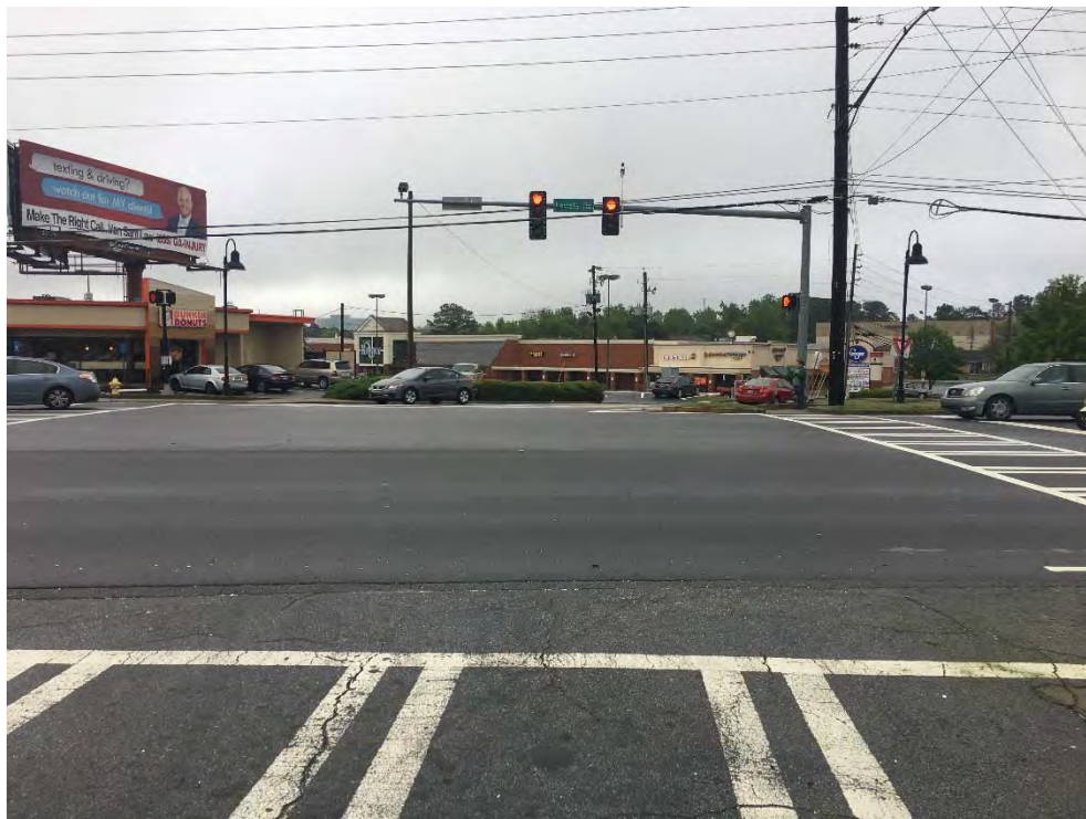
Figure A22: Southbound Approach, SR 236 at Montreal Road
