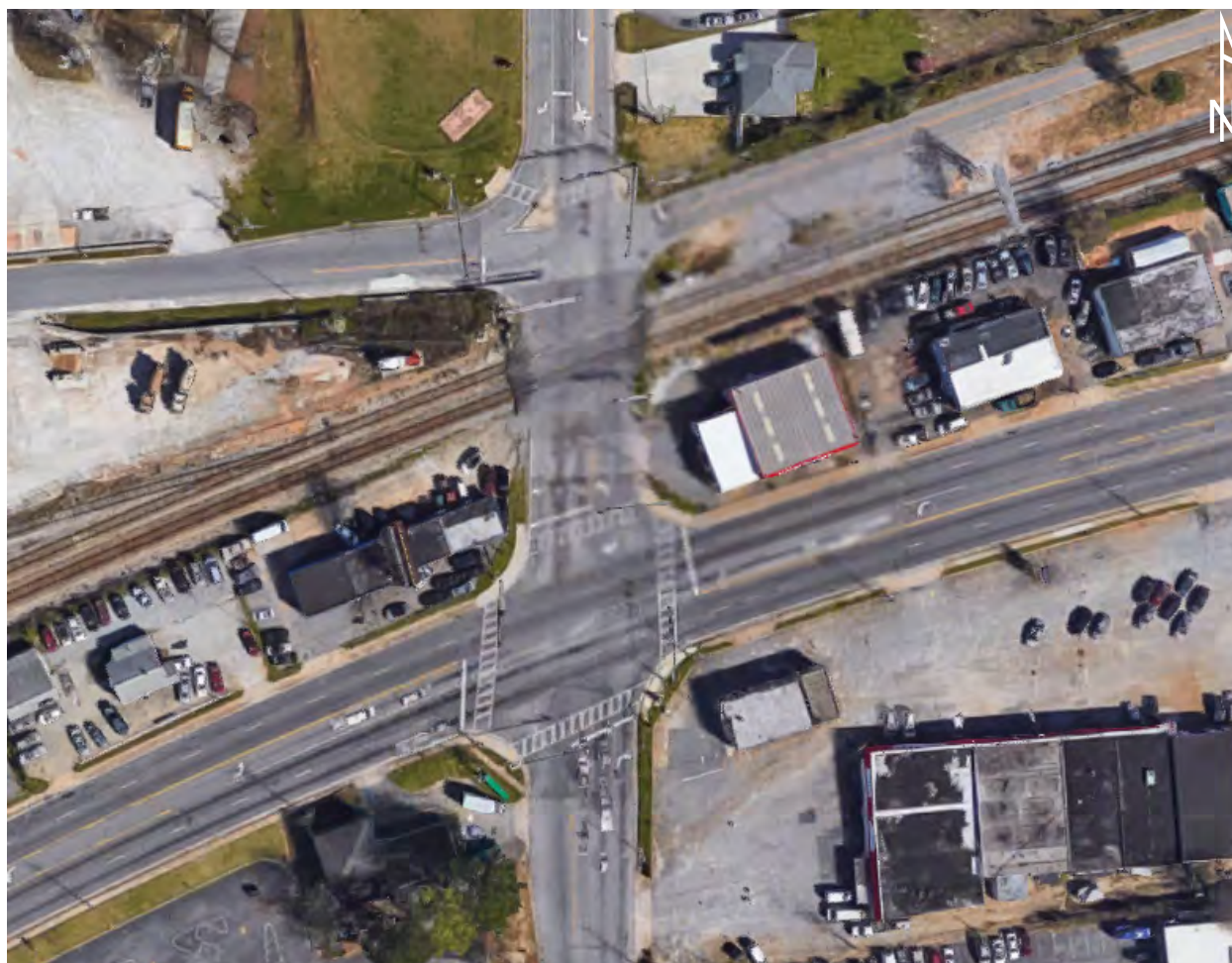
Figure 14: SR 8 at Brockett Road
