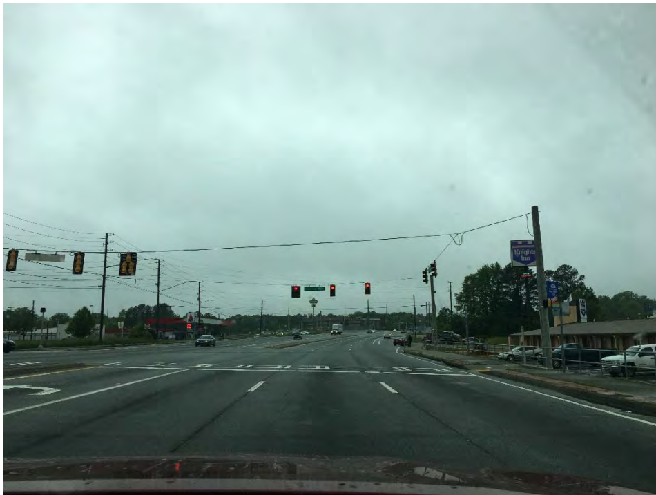
Figure A30: Westbound Approach, SR 8 at Montreal Road East
