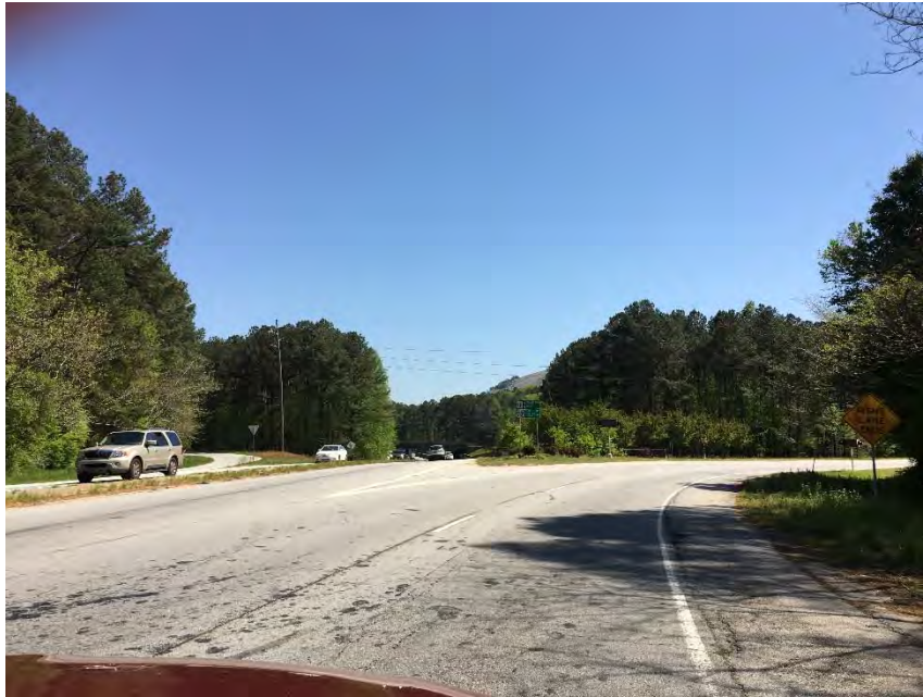
Figure A15: Southbound Approach On-Ramp, SR 10 at SR 236
