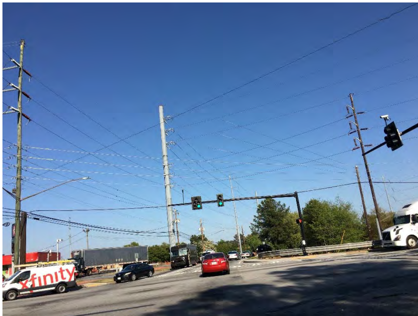
Figure A46: Eastbound Approach, Mountain Industrial Road at East Ponce de Leon Avenue
