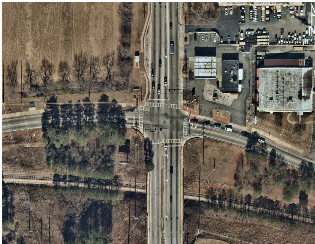
Figure 24: East Ponce de Leon Ave at Mountain Industrial Blvd/North Hairston Rd
