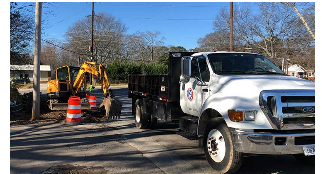
Downtown Tucker Streetscapes Phase II (Construction underway)
