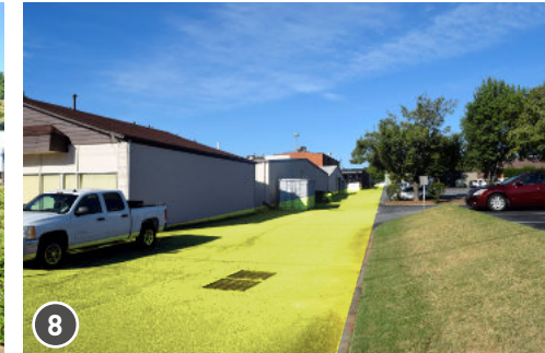
Block C, East-West Segment, adjacent to BOA parking
