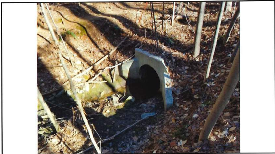
Photograph No. 2: Detention pond outlet on eastern boundary of project site.
