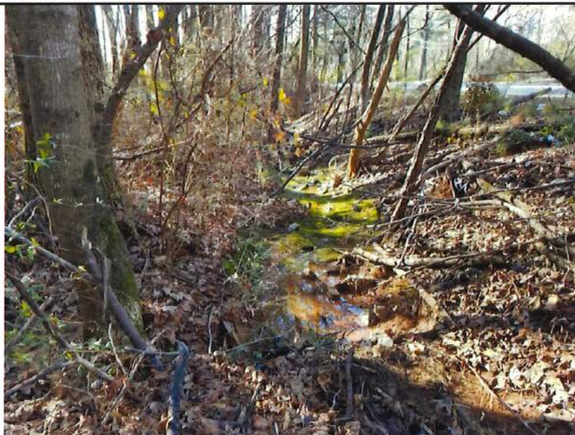
Photograph No. 4: Subject drainage feature in western portion of the site adjacent to Greer Circle.
