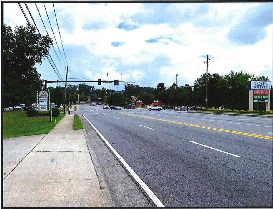
Photograph 1 – Lawrenceville Highway Facing North from Proposed RIRO Access Location
