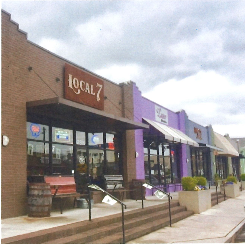
Figure 4- Building Complex Frontage on Main Street
