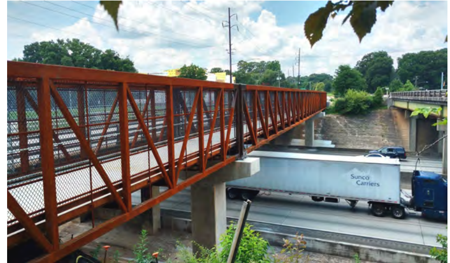
The Stone Mountain Trail pedestrian bridge over I-285 is located 5 miles south to Downtown Tucker
