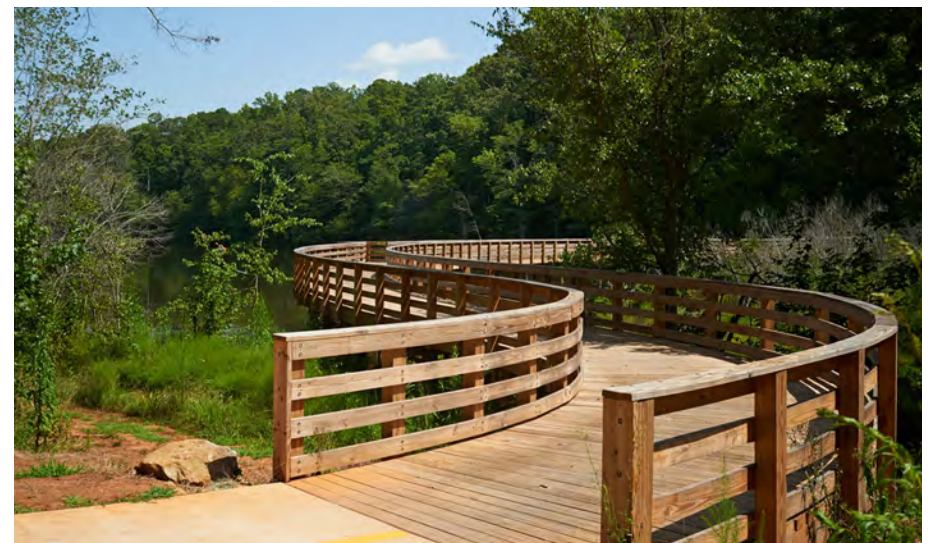
Wooden boardwalk structure for crossing lakes and wetlands.
