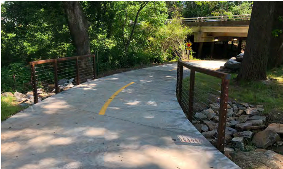
An example of the cable handrail with cor-ten finish
