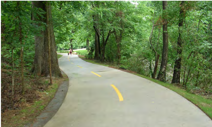
An example of incorporating the pervious concrete strip along the trail edge
