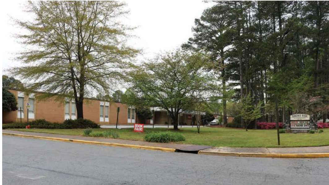
Figure 61. Smoke Rise Elementary School
