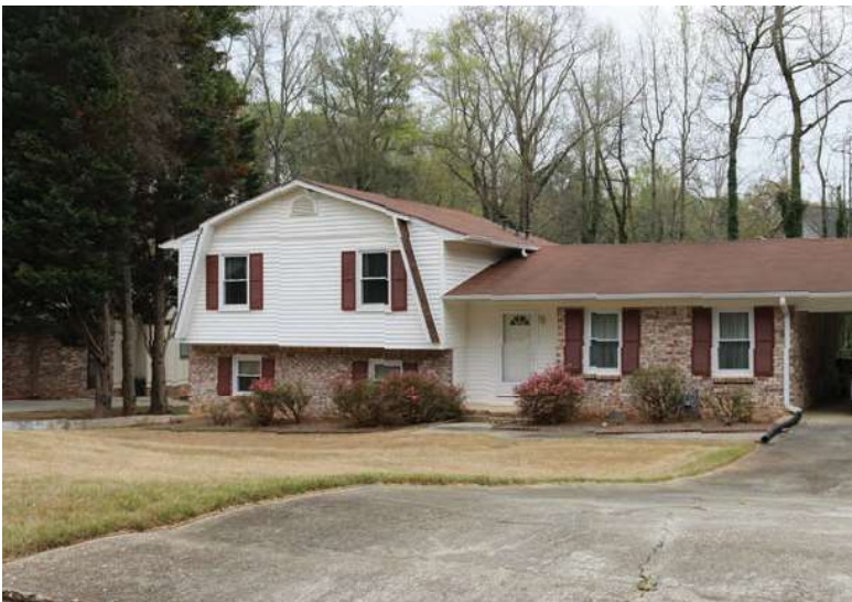
Figure 67. Plain Split Level with Gambrel and Gabled Roof, Drayton Woods Subdivision
