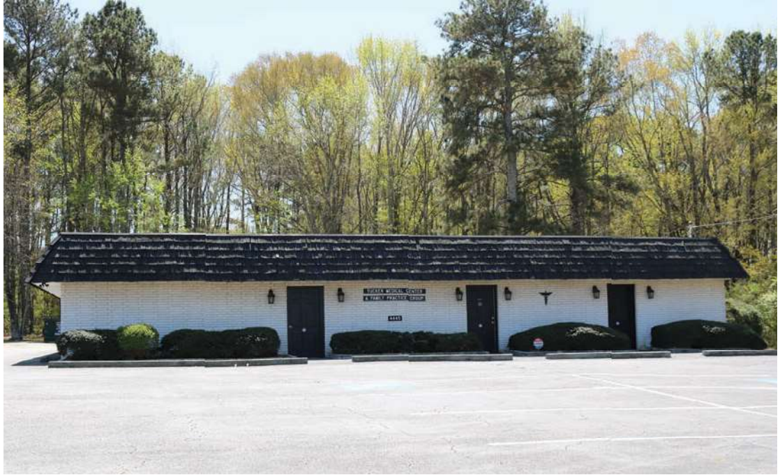
Figure 113. Historic Office Buildings, Cowan Road
