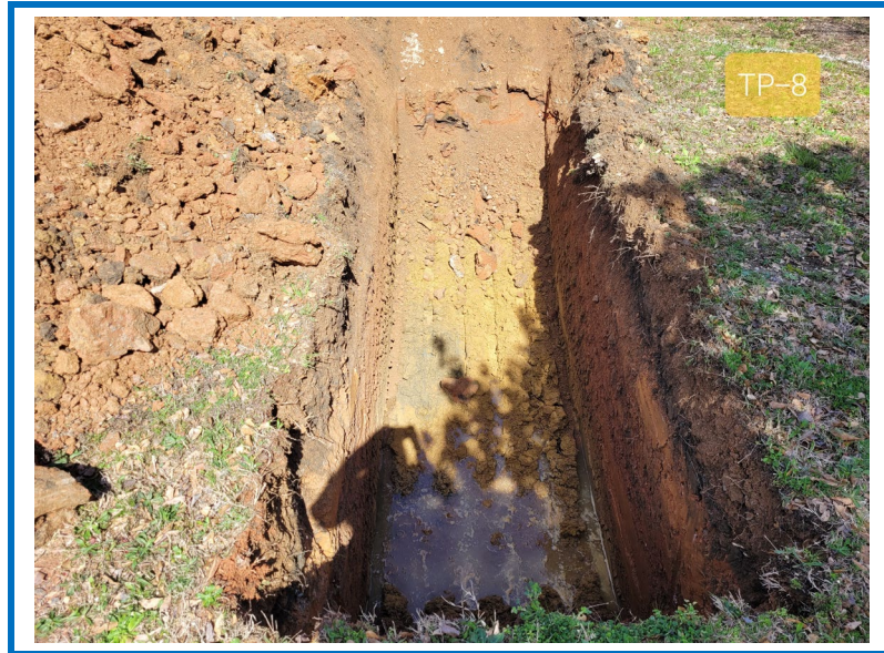
Photo 29: Test Pit TP-8
