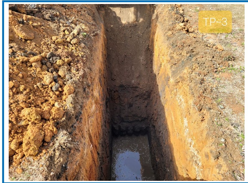
Photo 9: Test Pit TP-3
