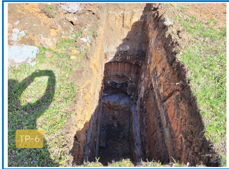
Photo 21: Test Pit TP-6
