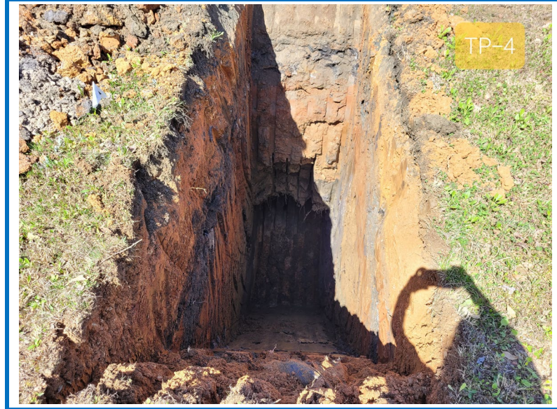
Photo 13: Test Pit TP-4
