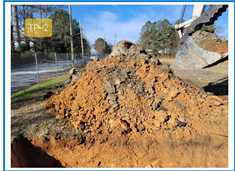
Photo 6: Excavated soils of Test Pit TP-2
