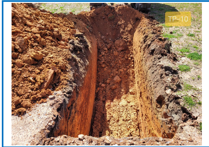
Photo 37: Test Pit TP-10
