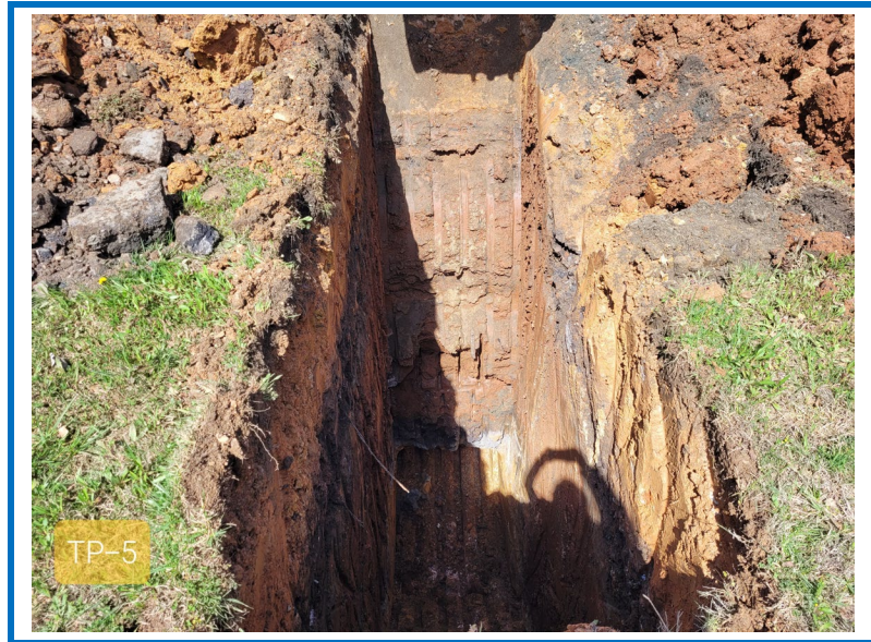
Photo 17: Test Pit TP-5
