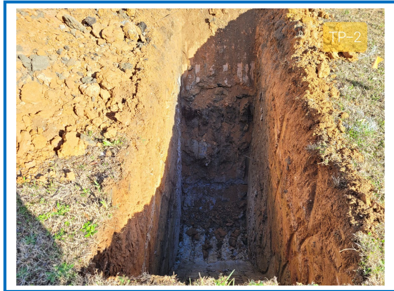
Photo 5: Test Pit TP-2
