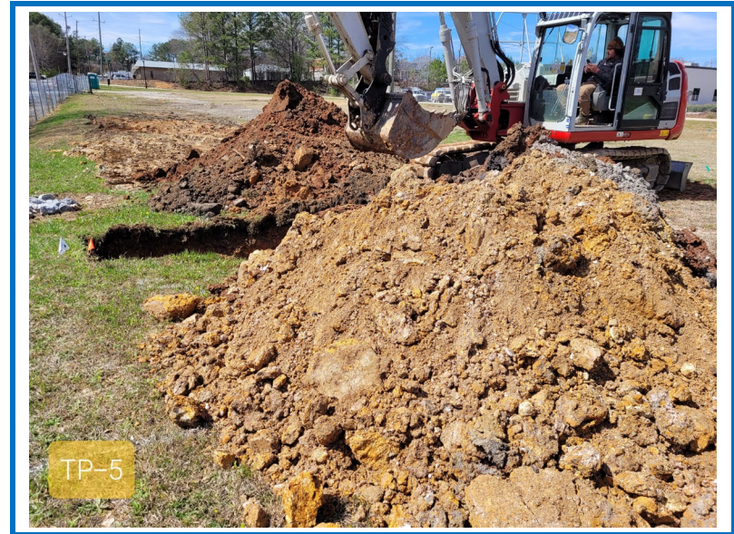
Photo 18: Excavated soils of Test Pit TP-5
