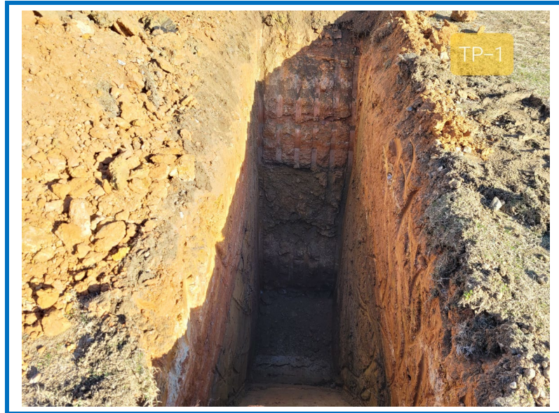
Photo 1: Test Pit TP-1
