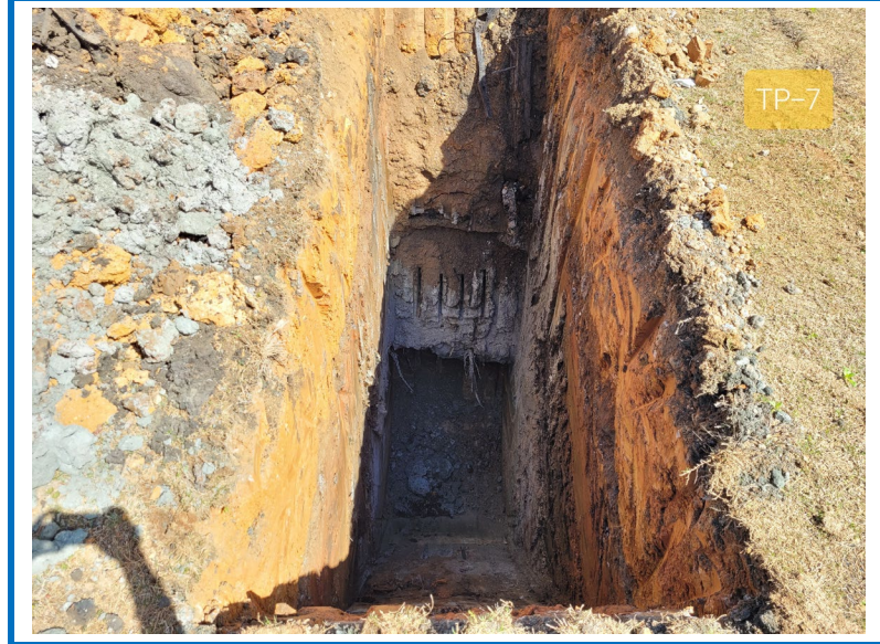
Photo 25: Test Pit TP-7
