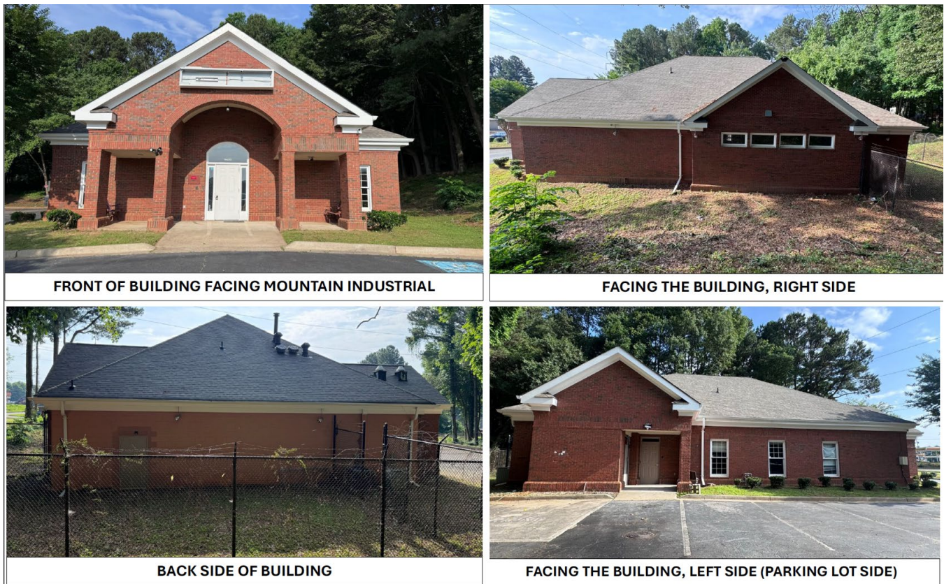
Figure 1. Building elevation photos (submitted by applicant).
