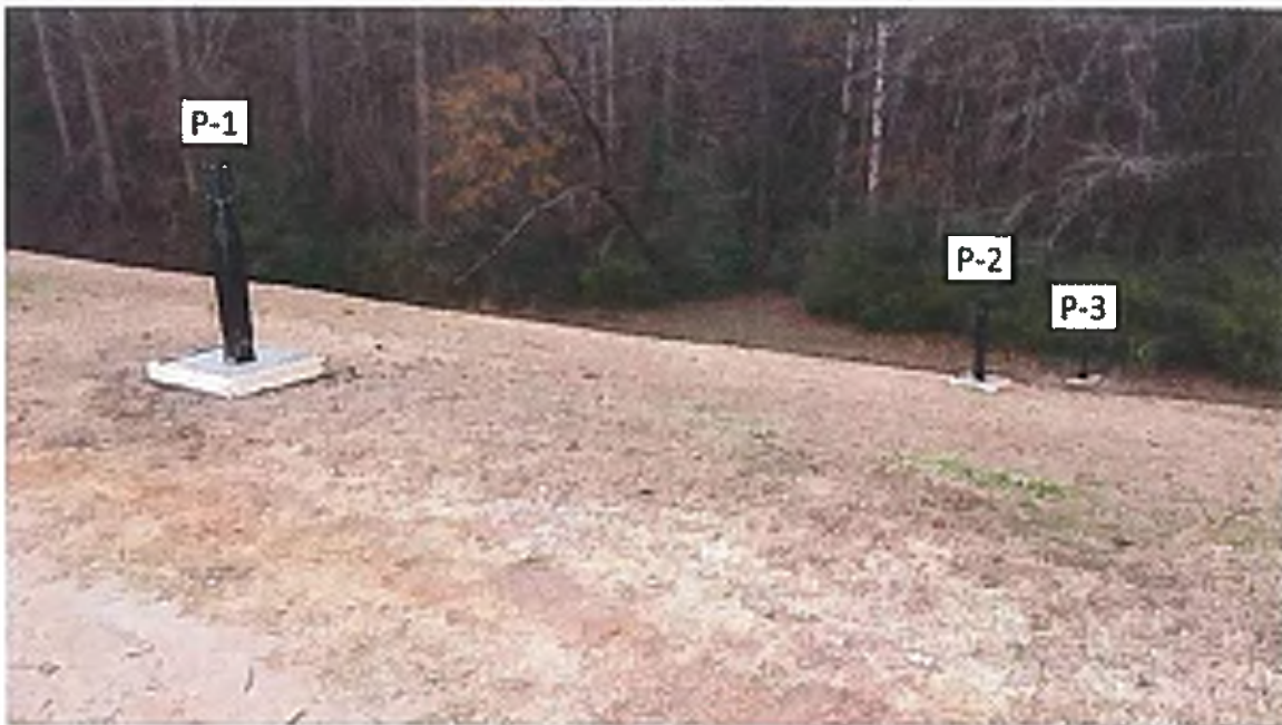
Piezometers P-1 through P-3; photographed on 12/6/2013
