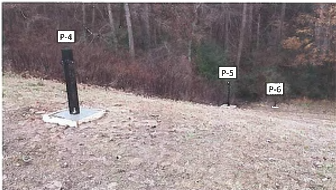
Piezometers P-4 through P-6; photographed on 12/6/2013
