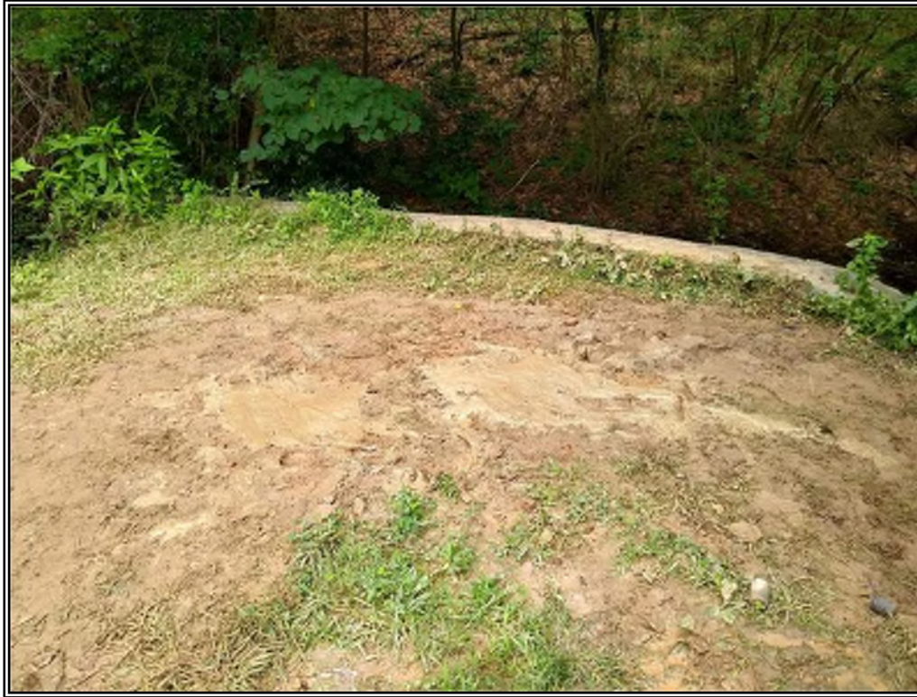
Showing boring AB-1 at the downstream area of the dam.
