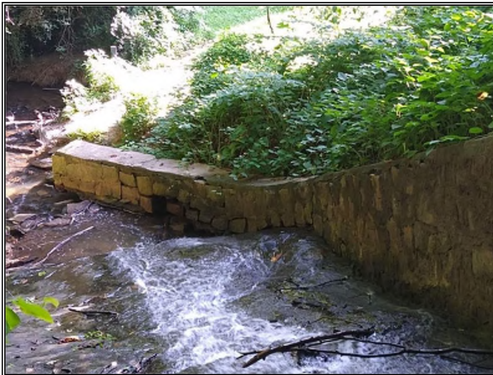
Old spillway located by the downstream face of the Dam.
