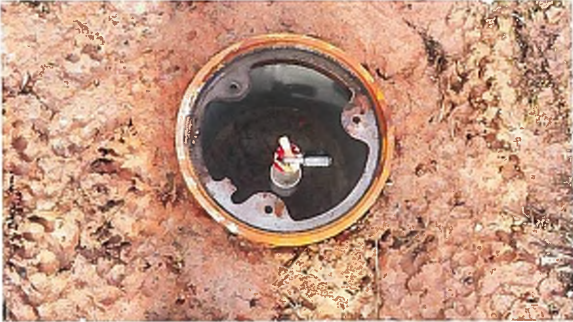
Repaired Piezometer P-4 with Protective Cover Removed; 01/27/2015
