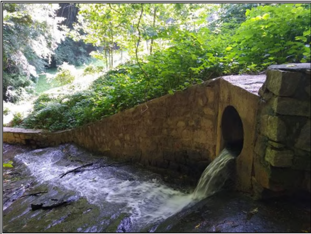
Concrete outlet located at the northern end of the left abutment.
