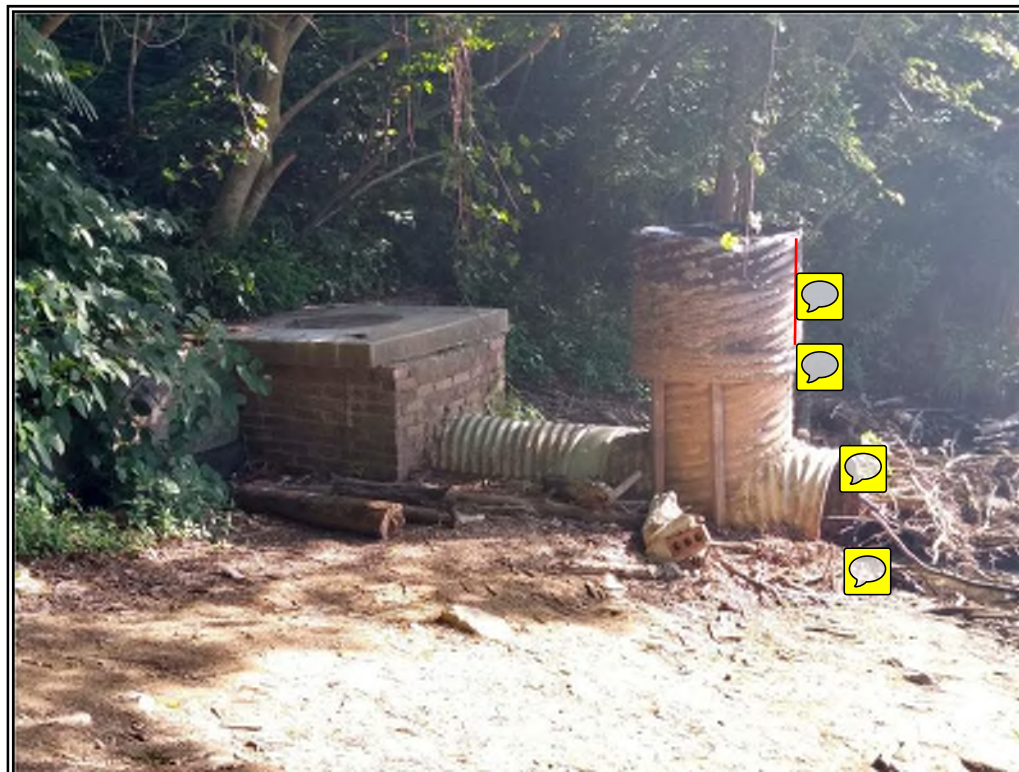
Spillway system located at the southwest end of the dam.
