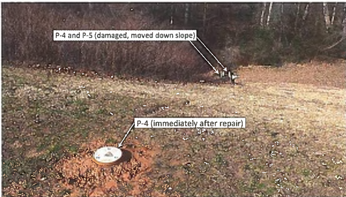
Repaired Piezometer P-4; Facing Northwest; 01/27/2015
