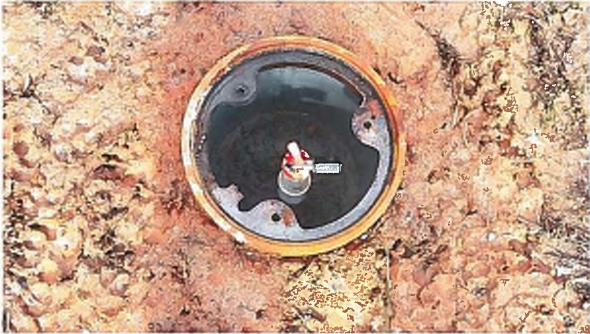
Repaired Piezometer P-4 with Protective Cover Removed; 01/27/2015
