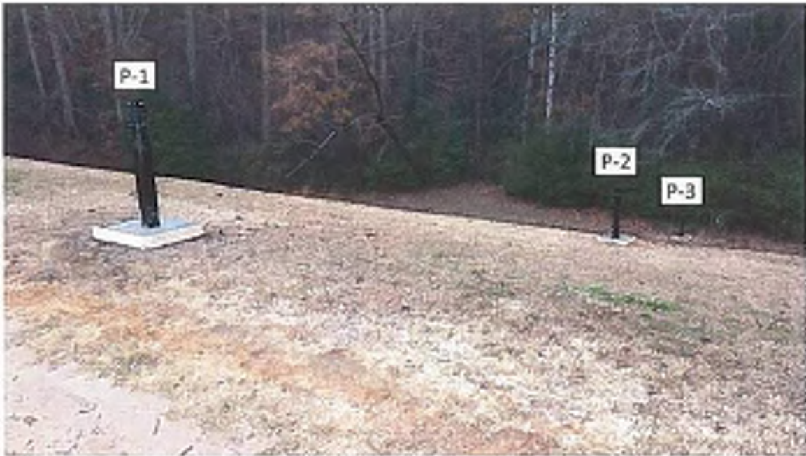
Piezometers P-1 through P-3; photographed on 12/6/2013
