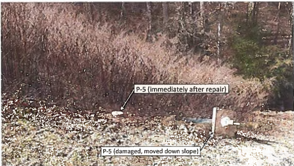
Repaired Piezometer P-5; Facing West; 01/27/2015
