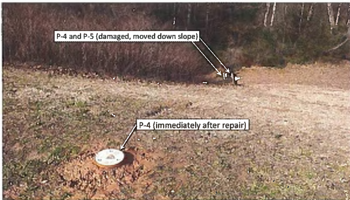
Repaired Piezometer P-4; Facing Northwest; 01/27/2015
