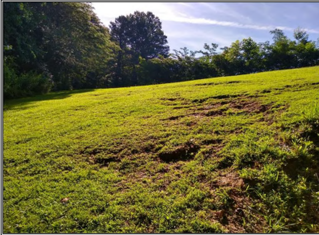
Site conditions from west of the dam looking east.
