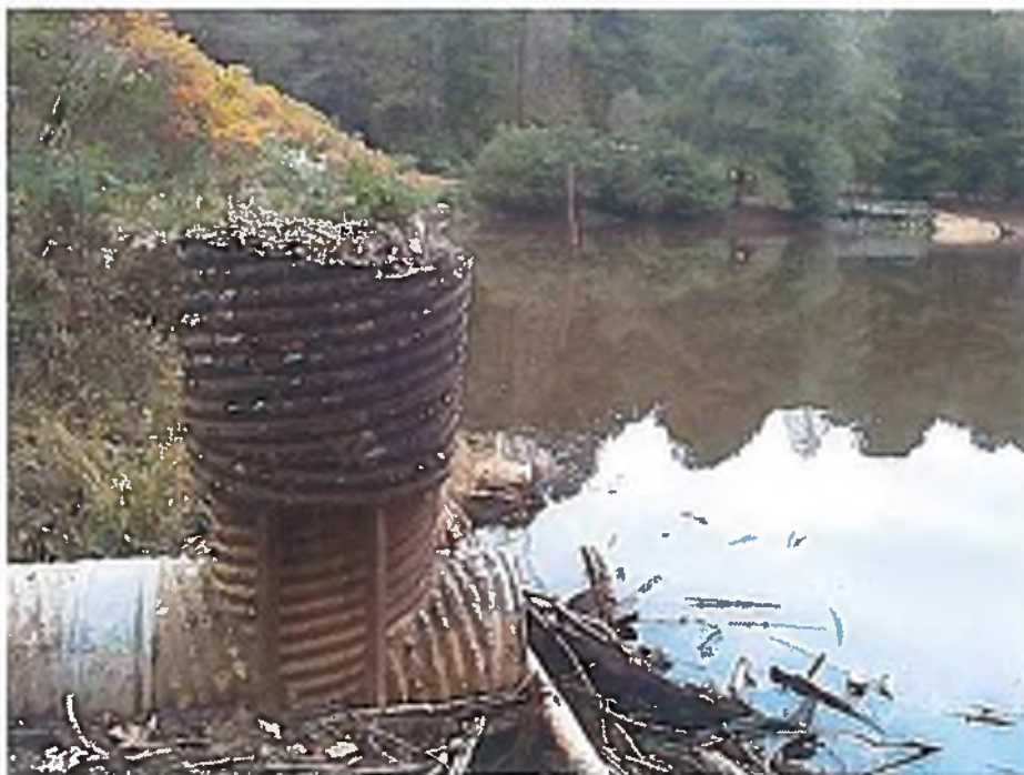
Principal spillway inlet and riser pipe; photographed on 10/28/2013
