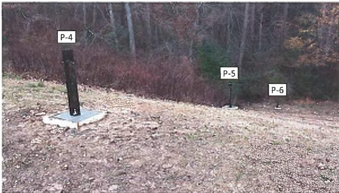
Piezometers P-4 through P-6; photographed on 12/6/2013
