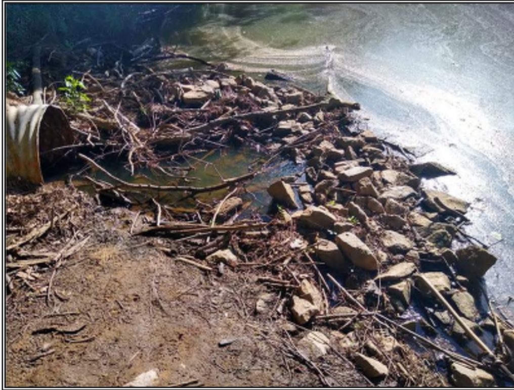
Outlet of the principal spillway constituted of riprap rocks.
