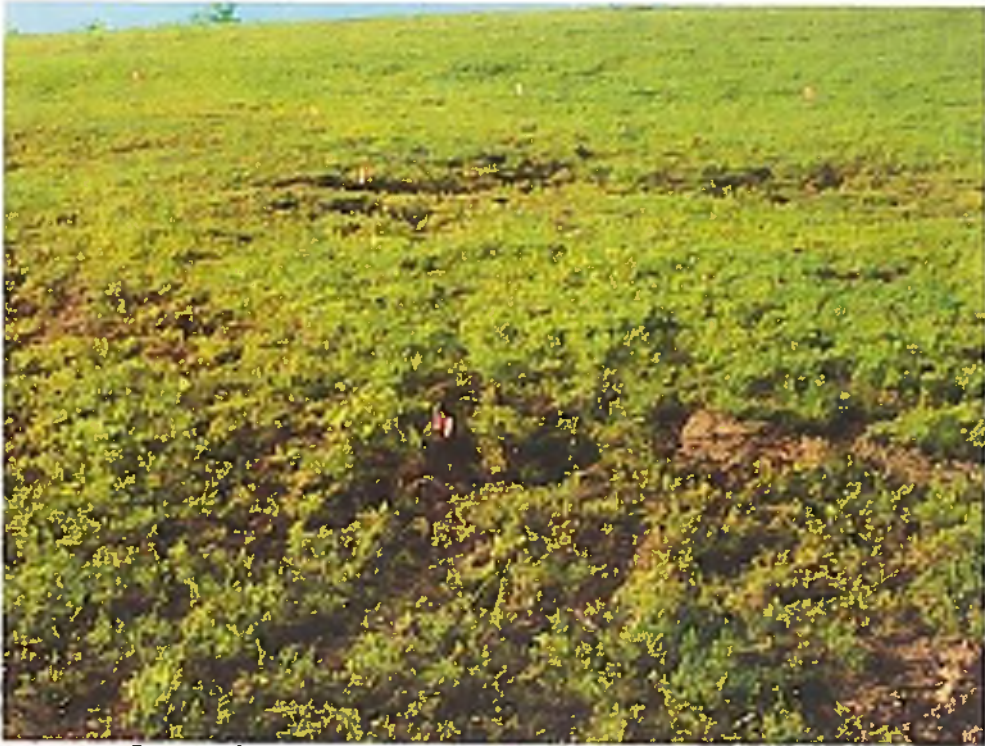
Smaller Slough Area – Downstream Slope, Erin Lake Dam
