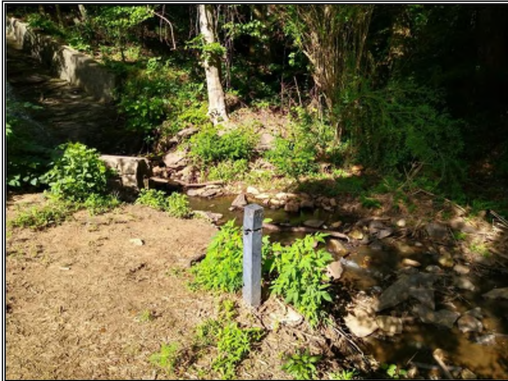
Downstream toe of the dam.
