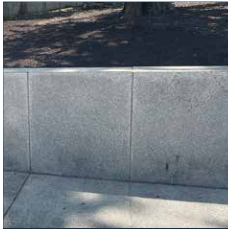
SITE WALL, CONCRETE
