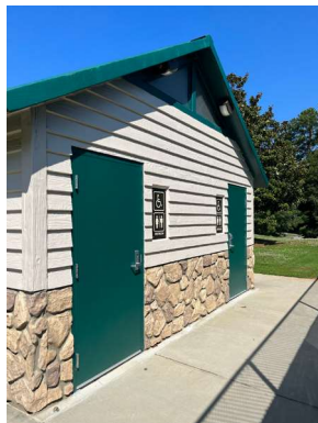
New restroom building
