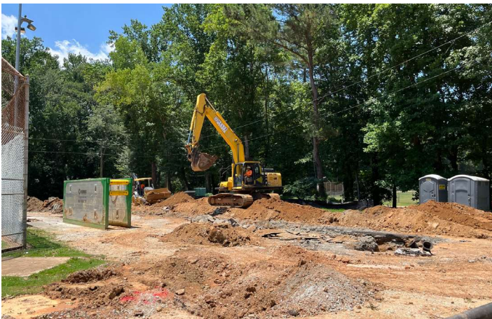
Site under construction during site visit
