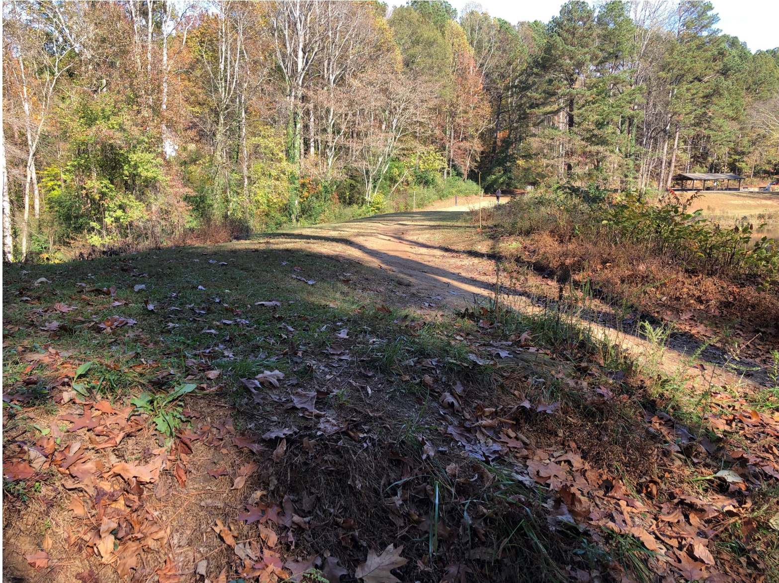
Vegetation on Slope of Dam
